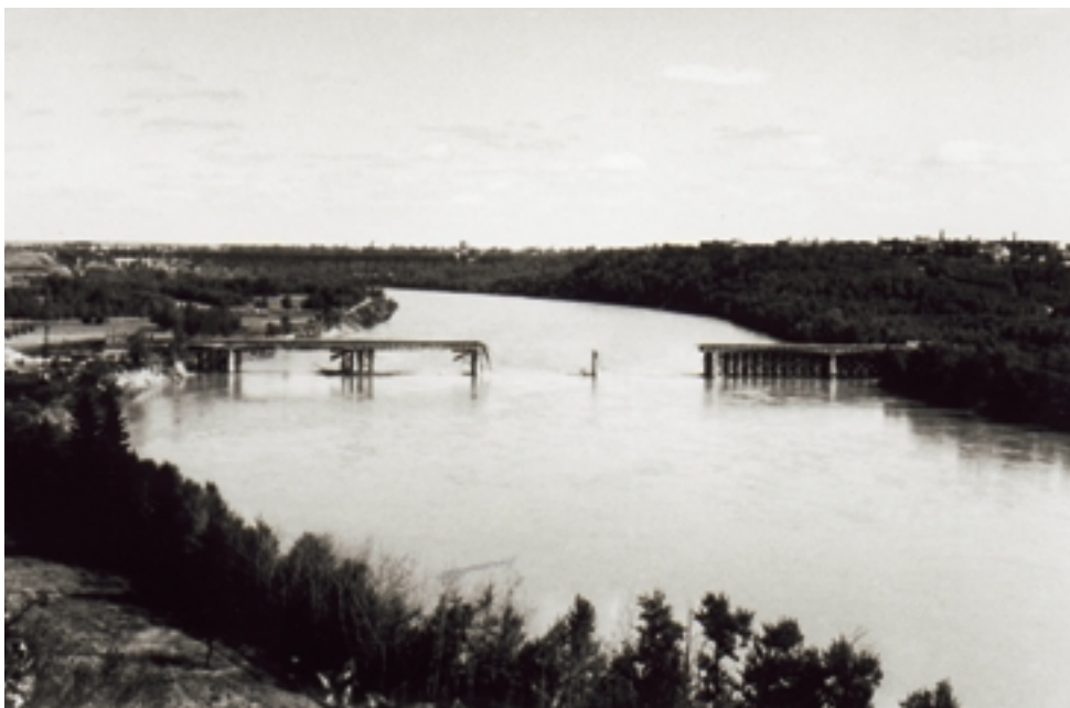
Figure 4.17 Edmonton's Groat Bridge was damaged by flood waters during construction.
